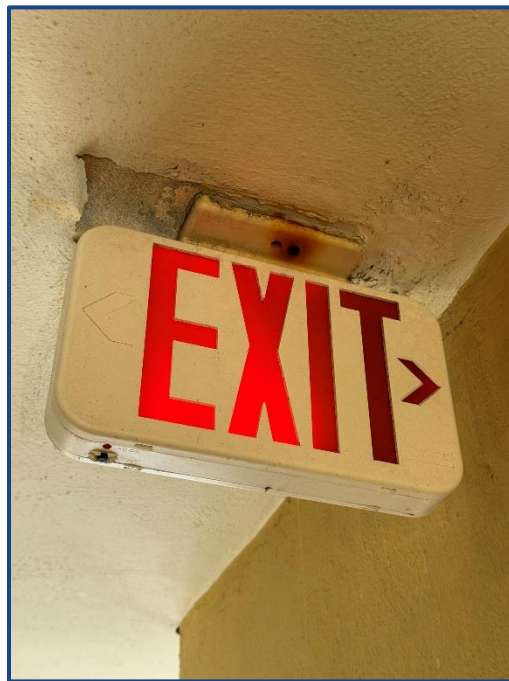
Photograph No. 18: Building Typical Fire Exit Sign
