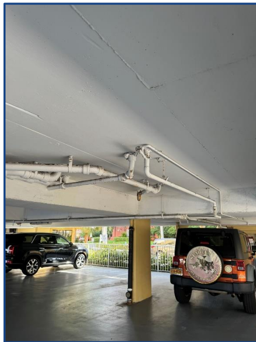
Photograph No. 10: Typical Building Parking Garage
