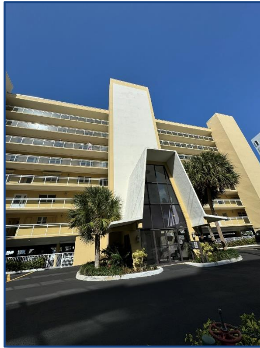
Photograph No. 3: Building East Elevation
