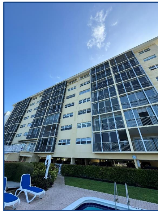
Photograph No. 2: Building West Elevation
