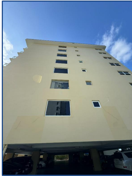
Photograph No. 1: Building North Elevation
