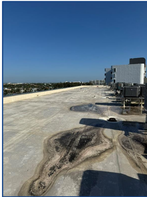
Photograph No. 6: Building Roof
