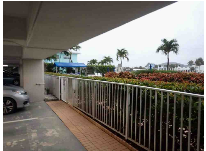
pool gates / perimeter fencing
