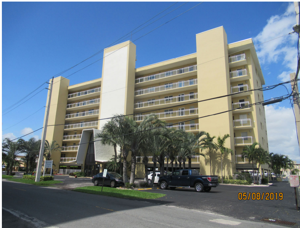
FRONT VIEW OF BUILDING
