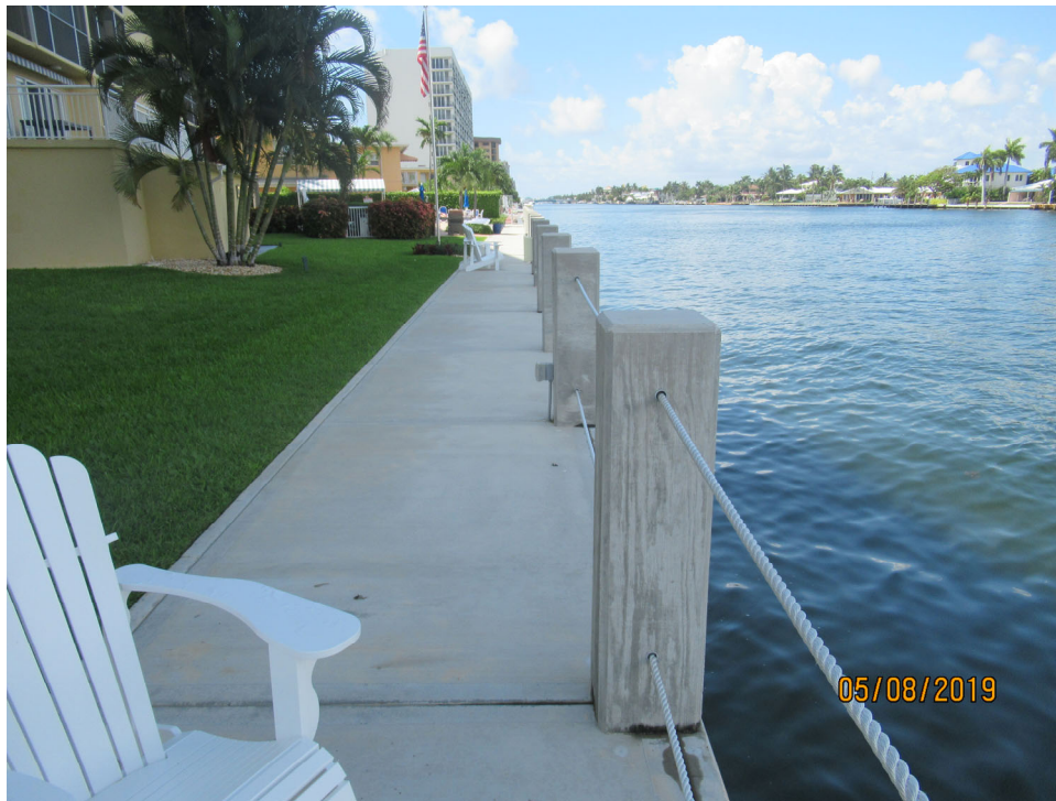
SEAWALL AND CONCRETE DECK
