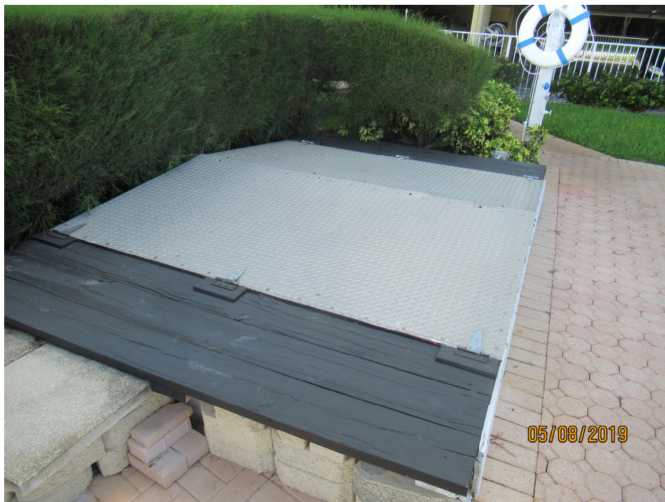
POOL EQUIPMENT SHELTER
