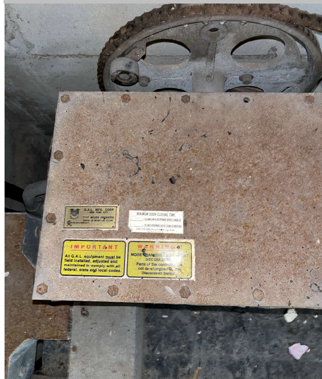
This is a GAL water resistant door operator. It needs cleaning and lubrication.
