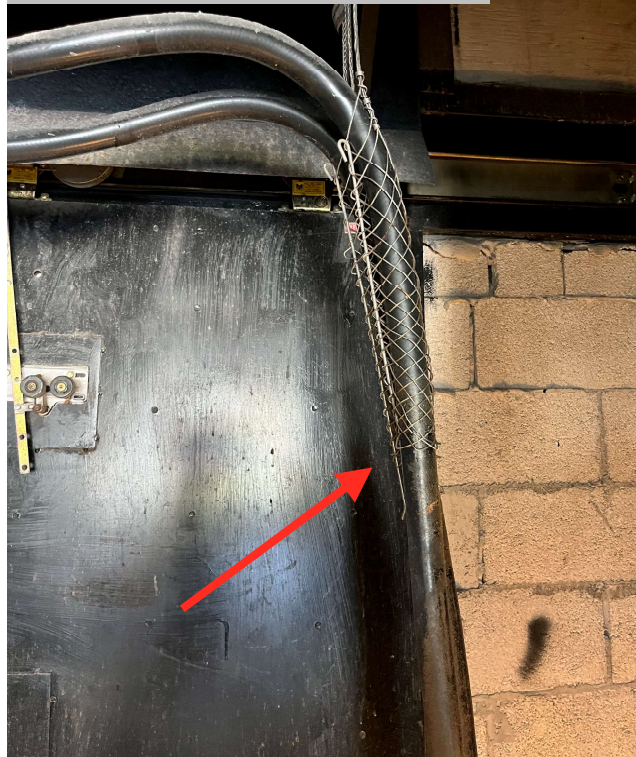
Kellum grip needs tape around bottom per manufacture.
