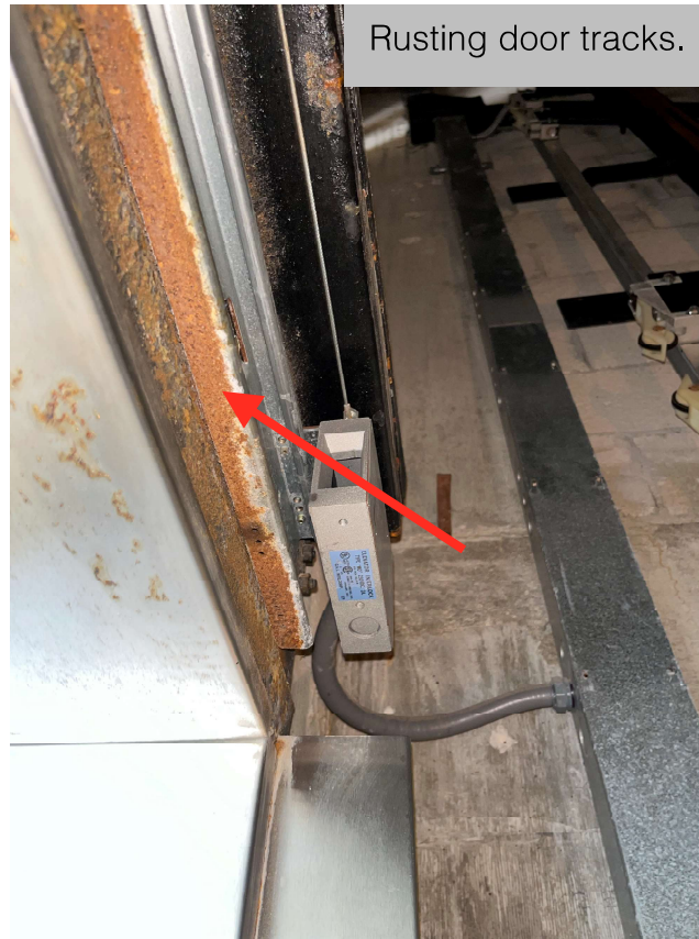
This is a GAL water resistant door operator. It needs cleaning and lubrication.
